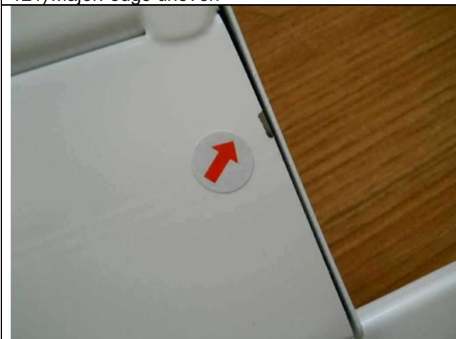
123) Major: poor coating
