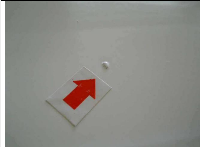
103) Minor: poor surface
