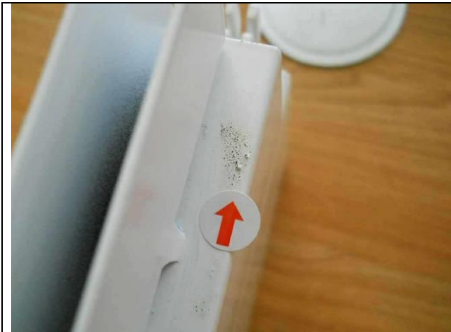
113) Major: poor coating
