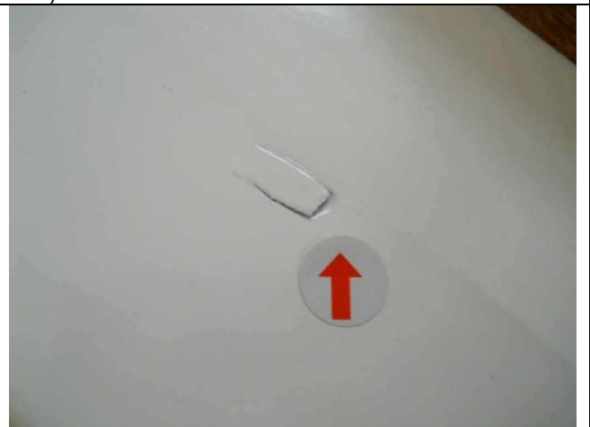
160) Major: poor surface
