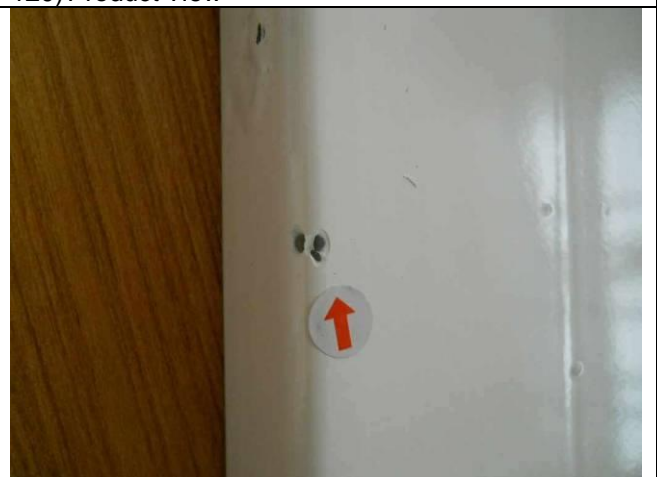
122) Major: poor coating
